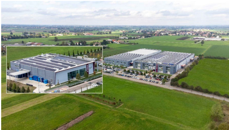
Innovation Center and expanded production plant in Caviago, Reggio Emilia, Italy
